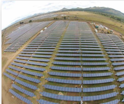
Witkop Solar Plant (30 MW), Limpopo
