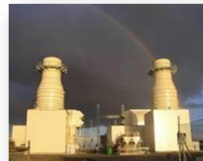
Ankerlig Power Station
