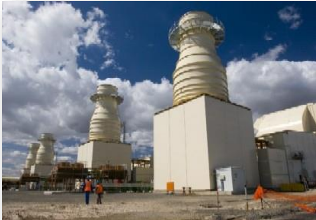
Ankerlig OCGT Power Station
